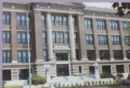
Our century old building has been a Kansas City icon in our Northeast neighborhood.
