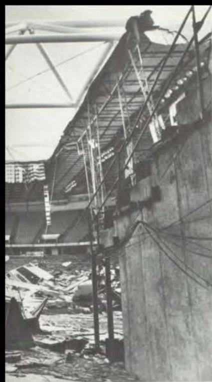
1. Kemper Arena was damaged during a heavy rainstorm June 4, 1979. The building was used to stage concerts, the American Royal and the Kansas City Kings basketball games. 2. Buying her ticket for the RUSH concert, from Second Coming, senior Ceresa Hall prepares to go to Kemper Arena after it was rebuilt. (photo 1 by Duane Woner, courtesy of the Examiner; photo 2 by John Capp)
