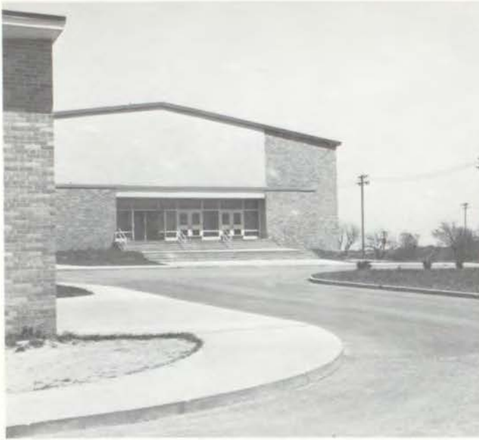
The spacious circular driveway facilitates the elimination of some of the traffic problems at Beartowns and the many football and basketball games held on Chrisman's field and in its school gymnasium. It also provides adequate parking space for visitors during the day.
