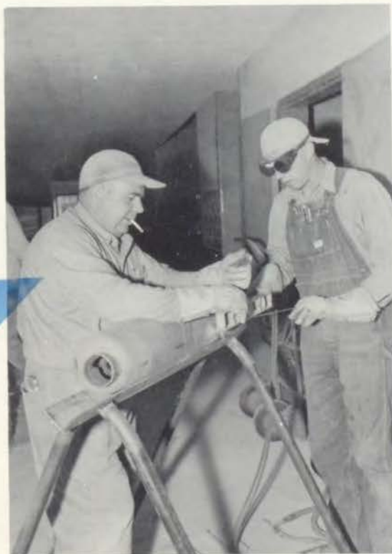
Construction workers who are striving dilligently for completion of facilities.
