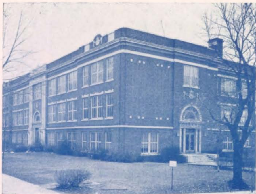
William Chrisman High School Built in 1916 West Entrance
