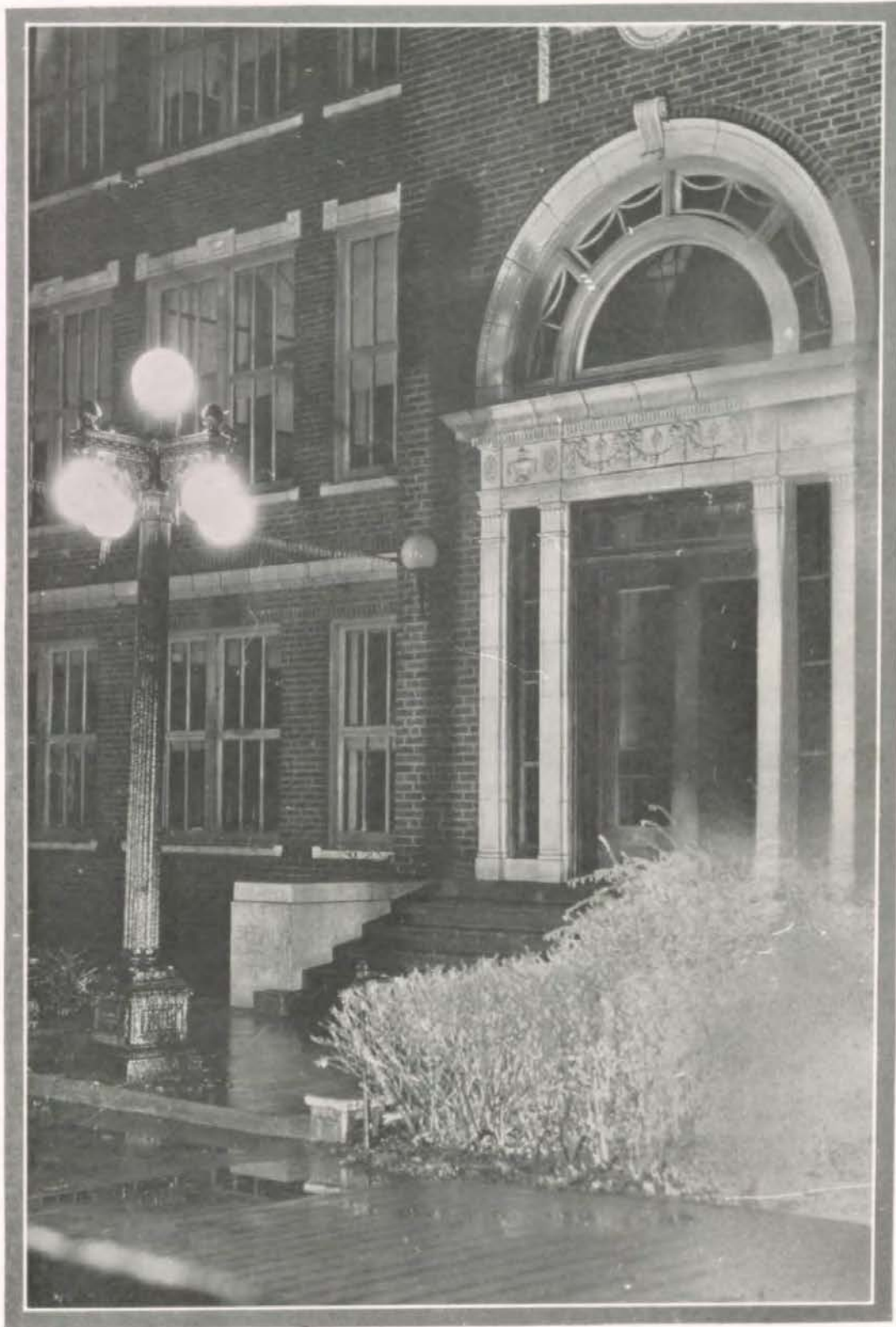
EAST ENTRANCE BY NIGHT
