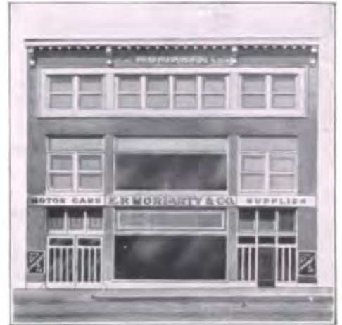
Our New Building
