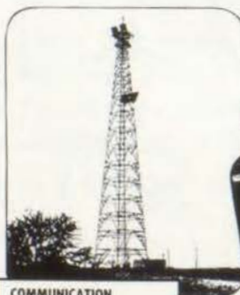
COMMUNICATION 350 Ft. Self-Supporting Micro-Wave Relay Tower for Television and Telephone Transmission
