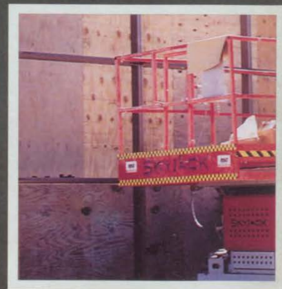
Above: The Goppert Center under construction, summer 2001.
