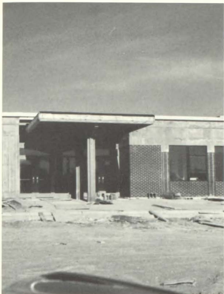
Smith-Hale under construction May 1968.
