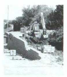
A retaining wall is being painstakingly rebuilt after imperfections in the original construction caused concern about safety.
