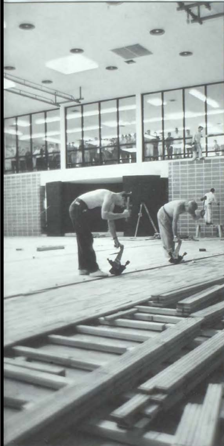
The revolutionary 'floating floor' being installed in 1962.
