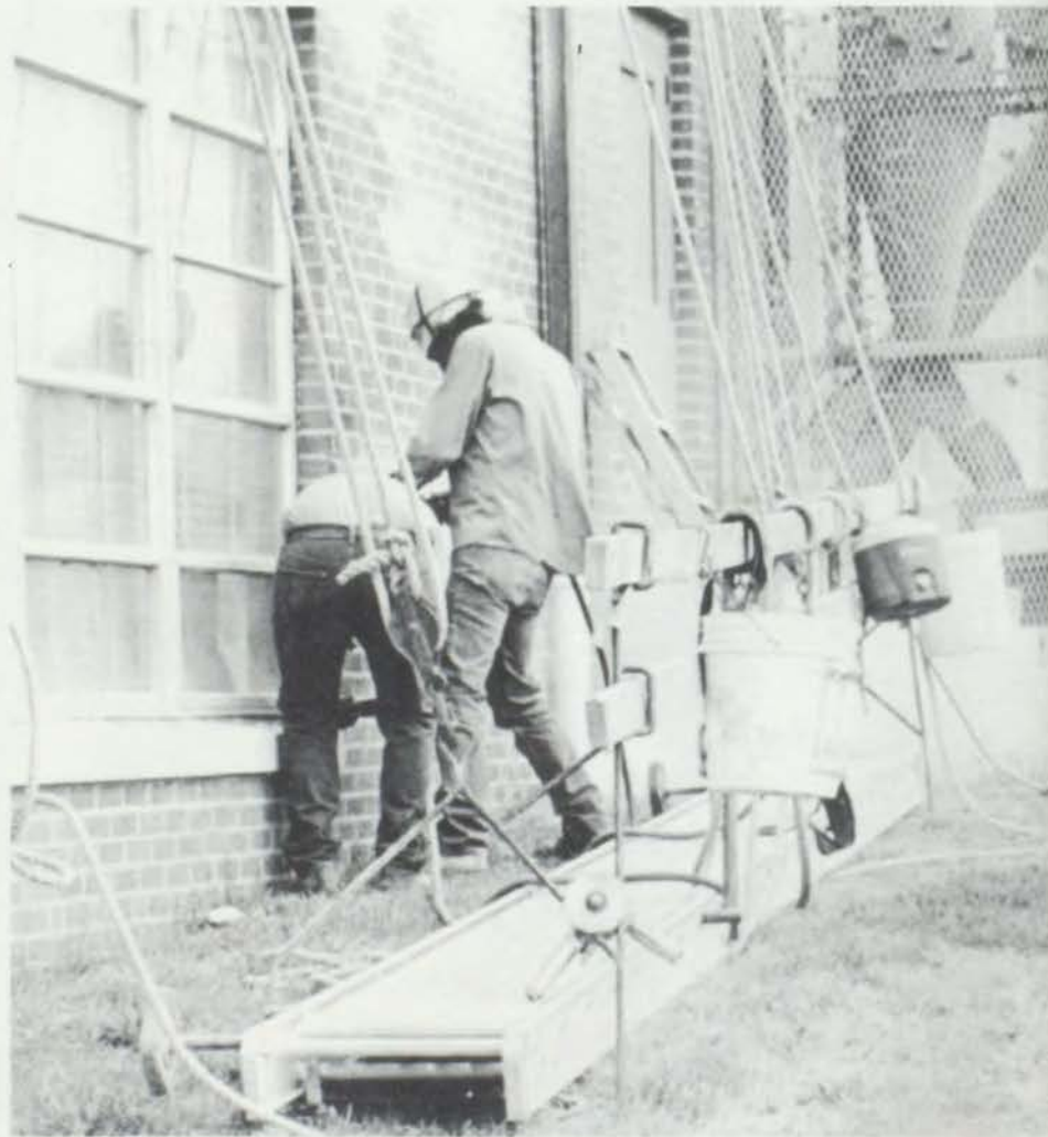
Two construction workers "tuckpoint" on the east side of the building. The work was conducted before, after, and during classes in September.
