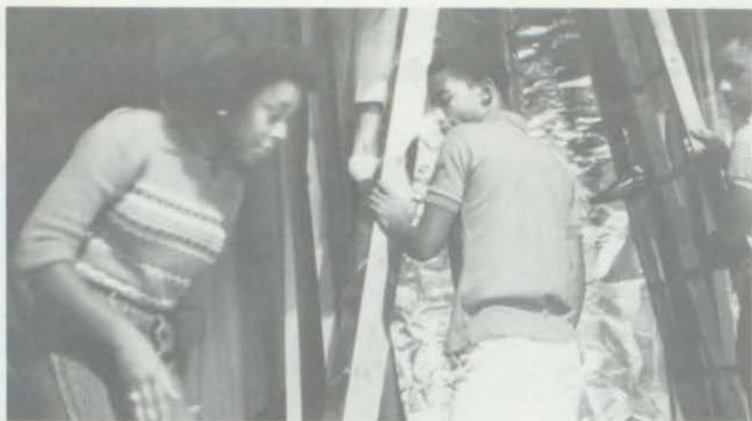
The road to progress is always under construction.
