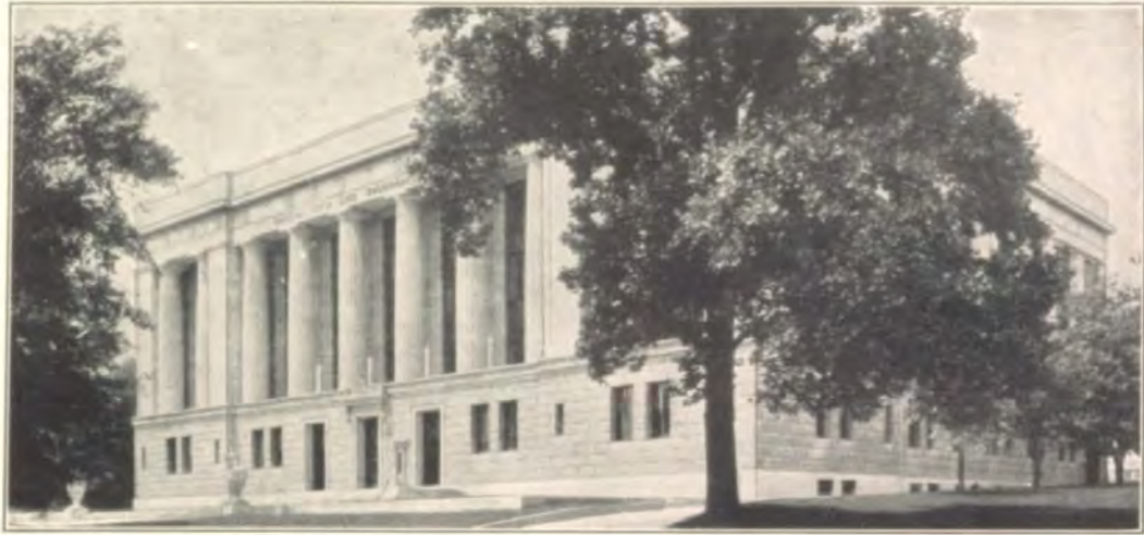
Home Office Building 3520 Broadway
