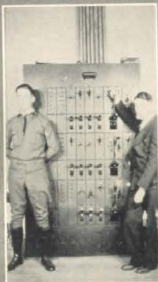
STAGE SWITCH BOARD
