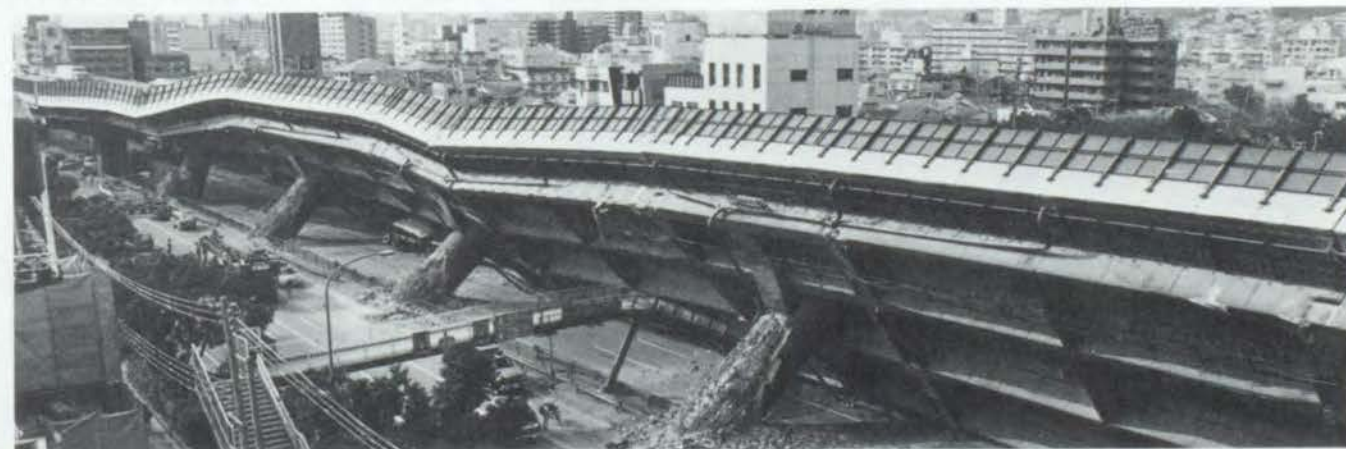
A highway bridge is knocked over in downtown Tokyo after a recent earthquake. Regions of Japan are ripped apart each year by the destructive powers of earthquakes.
