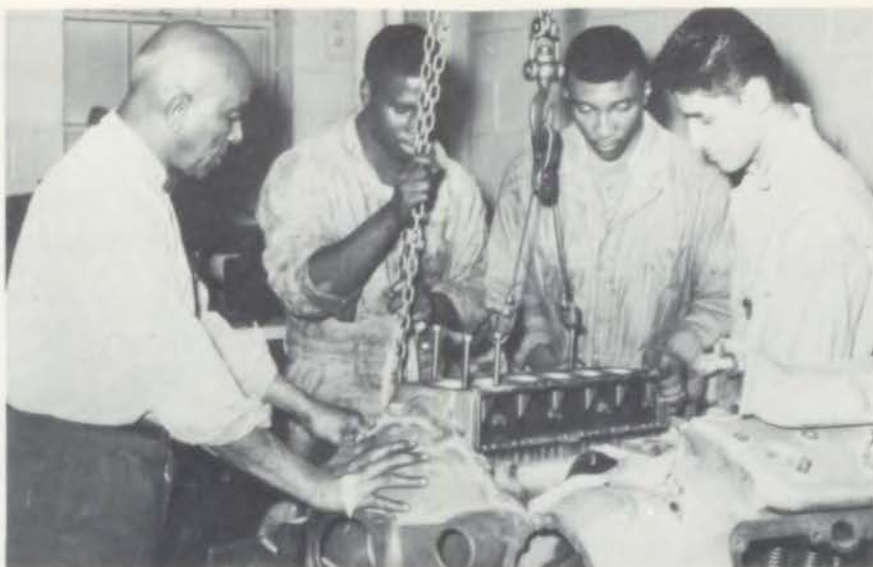
James Polk, Rennie Gordon and Felipe Fernandez demonstrate their mechanic skill in overhauling a Ford six engine. Mr. Russell evaluates their technique.
