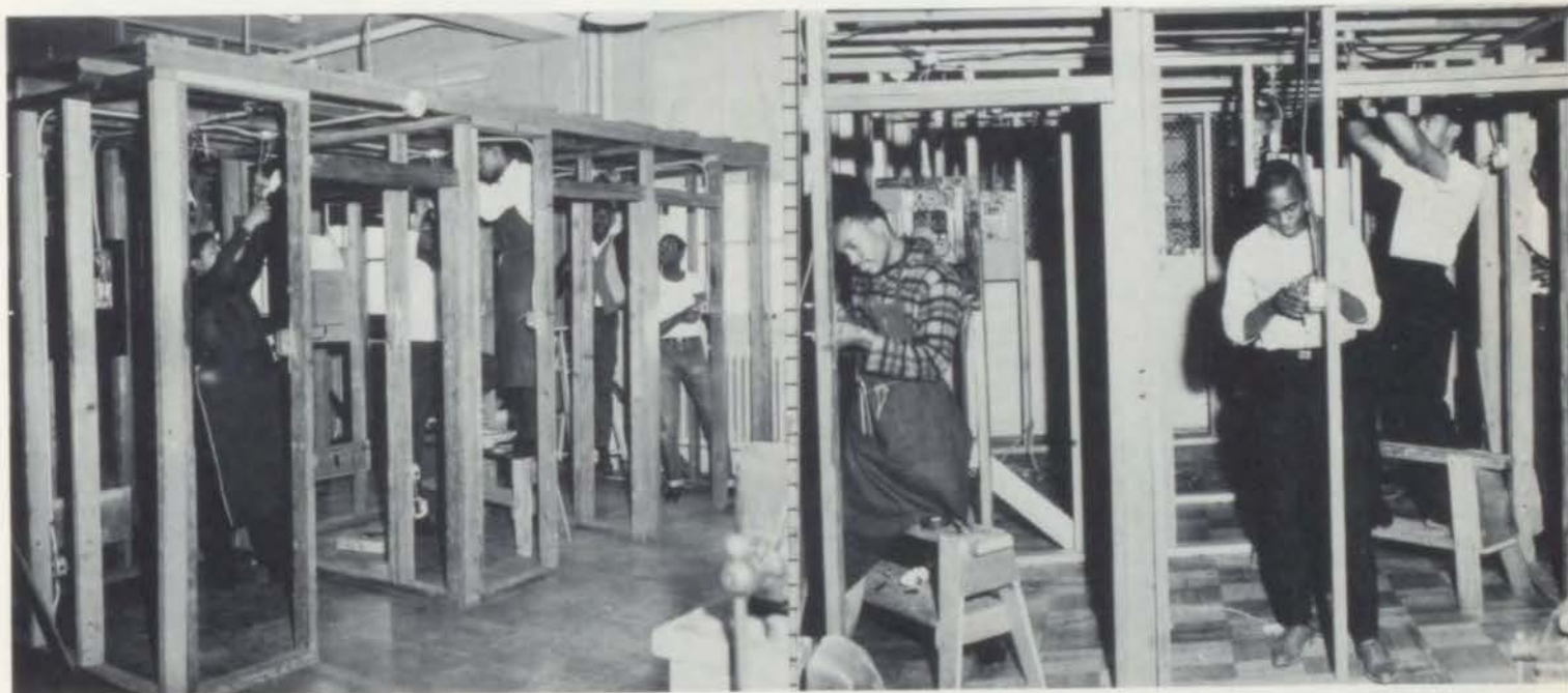
These students are putting the final touch on their wiring booths. Their major area of interest is Interior House Wiring. Each boy hopes his job will meet the high standards set by his instructor Mr. Stewart.
