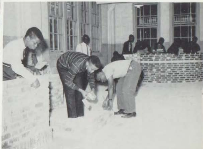
From Left To Right; Ronald Scott is building a garden wall, Gene Robinson is starting a common bond corner. The rest of the class is working on a half circle femish bond with a dental head. Lawrence Downton, in the center, checks the work.
