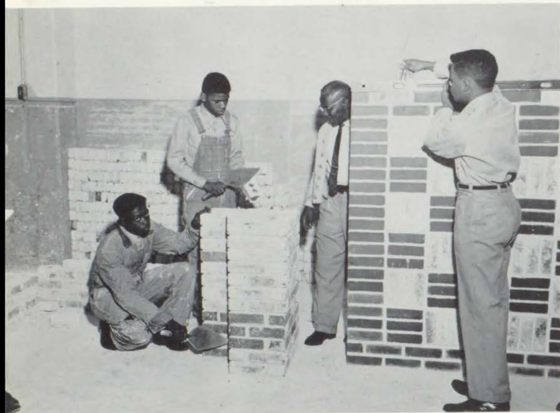
These students are working on different projects and designers from Left To Right; Roosevelt Gipson and Jerry Lark working on an L pier. Mr. Smith, instructor, looking on and John Bennett working on a basket weave.
