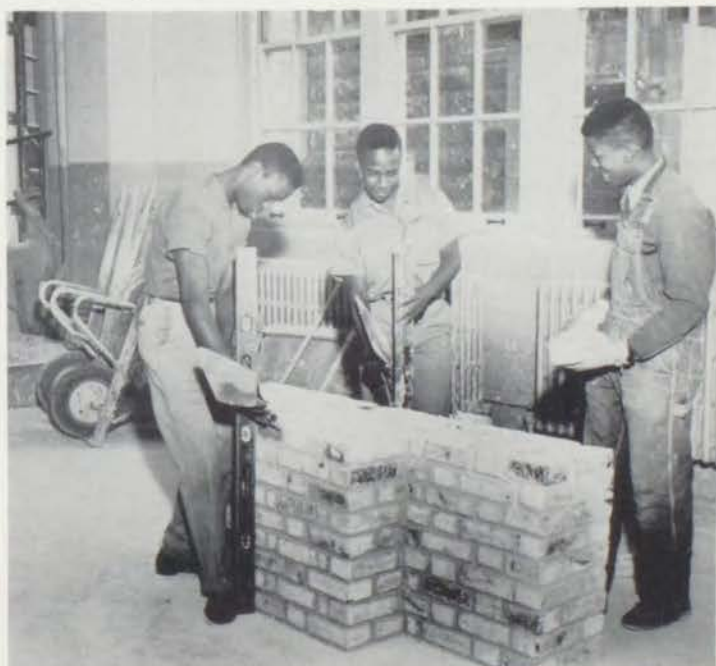
Willie Ferguson and Jerry Lark working on a femish bond wall with an 8' x 21' pilaster.
