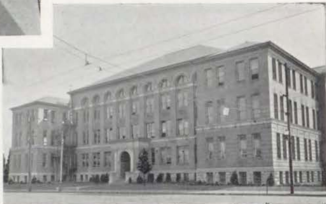
The North building from Fifteenth street.
