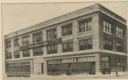
OUR NEW COLLEGE BUILDING.
