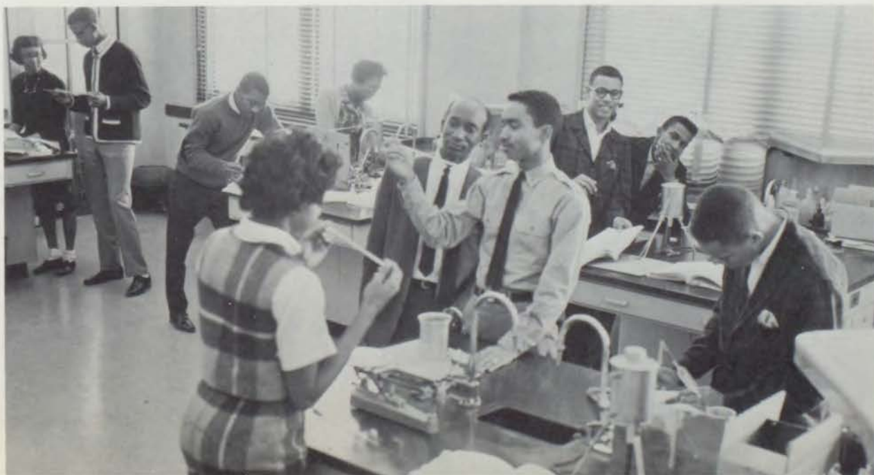
Mr. Darton, Physics instructor, is inspecting a centigrade thermometer as these students perform an experiment to determine the specific heat of a metal.
