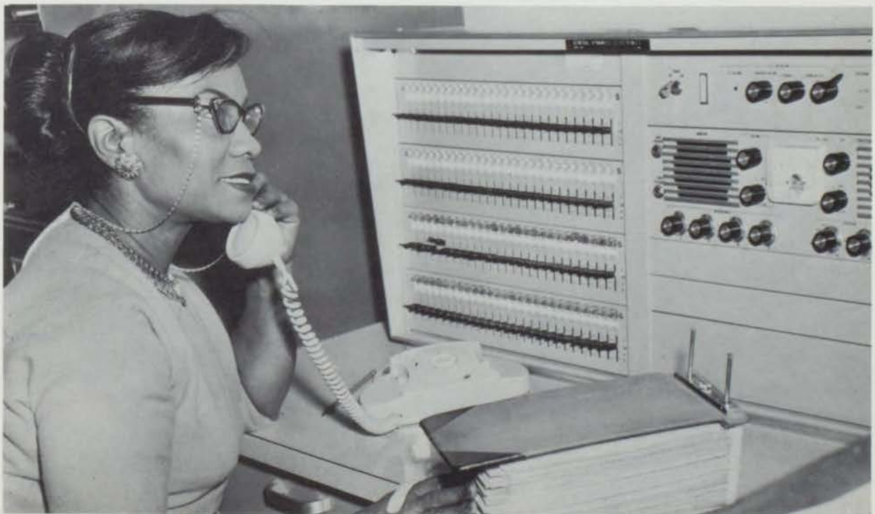
MRS. HUGHES operates Intercom switchboard.
