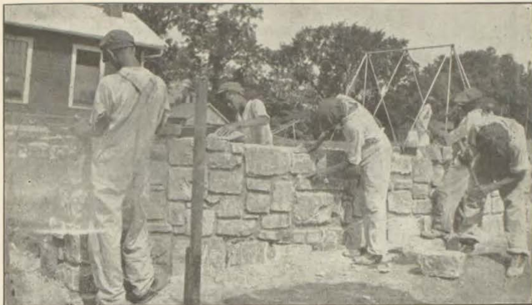
MASONRY BOYS LAYING FOUNDATION OF ATTUCKS SCHOOL ANNEX.
