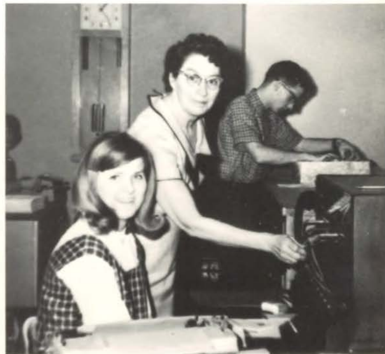
(right) Linda Booton and Mrs. Martin at the office switchboard. The people in the office training program put in a hard day's work while gaining important information that will aid them after graduation when they go on to other jobs.
