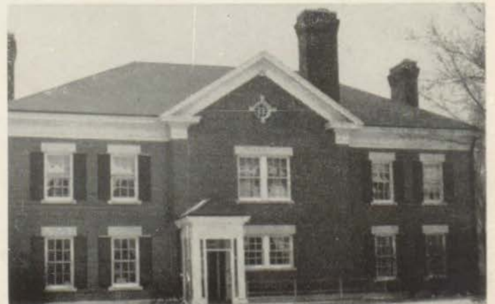
This building is one of the two dormitories. It houses the younger boys, the central heating plant, the kitchen, and dining room.
