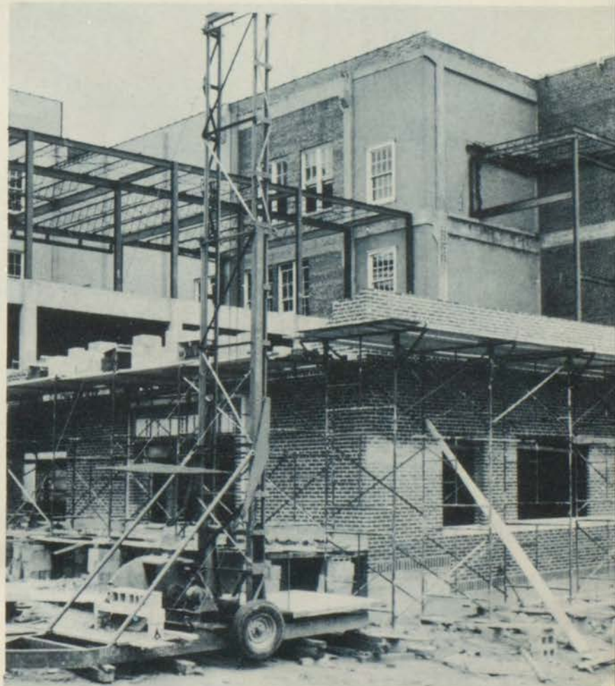
Viewing construction of the long-awaited girls' gym.
