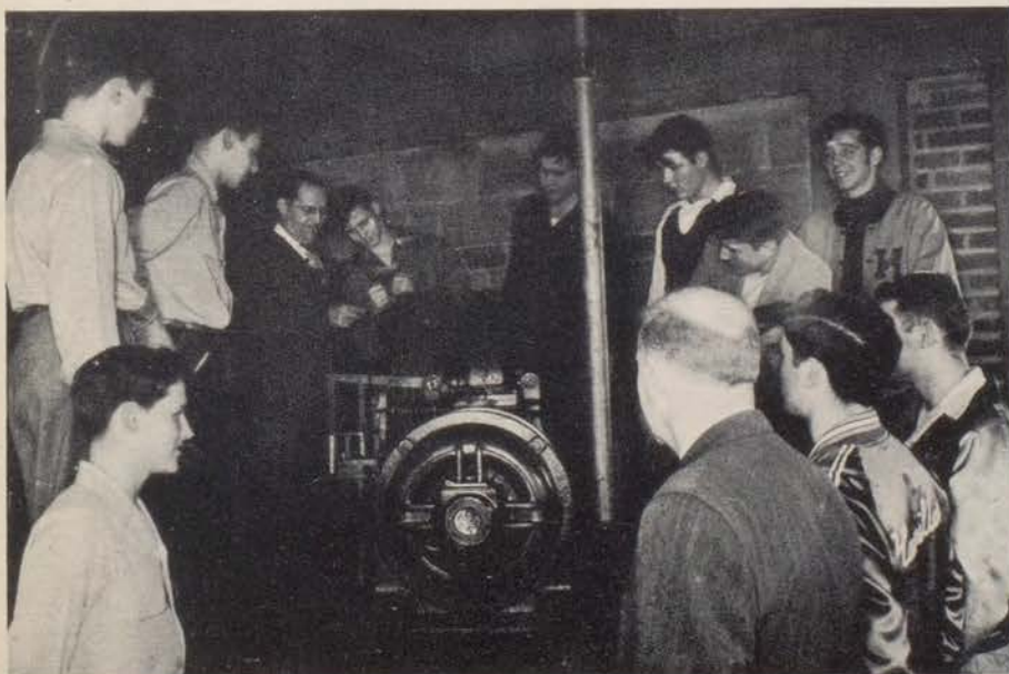
Inspecting the mechanics of the elevator shaft.
