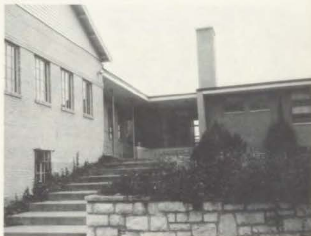
Front view of Vaugirard, CBC's own retreat house.
