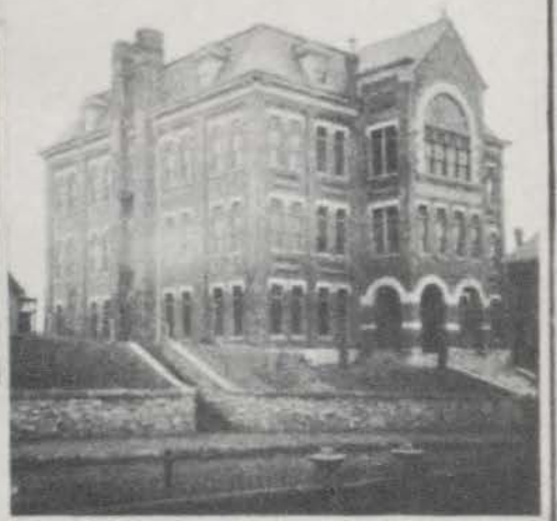
PRESENT BUILDING COMPLETED IN 1892.
