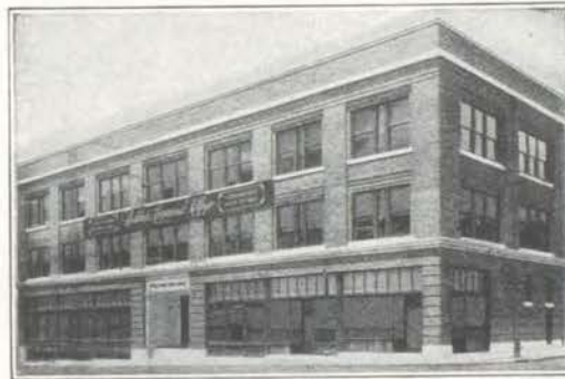
OUR NEW COLLEGE BUILDING.
