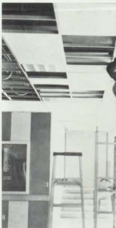
▶ Over the summer workers replaced old ceiling tiles with asbestos free ones, done in preparation for the new school year. Here tiles are being replaced in front of the auditorium. Photo: Michelle Blaser
