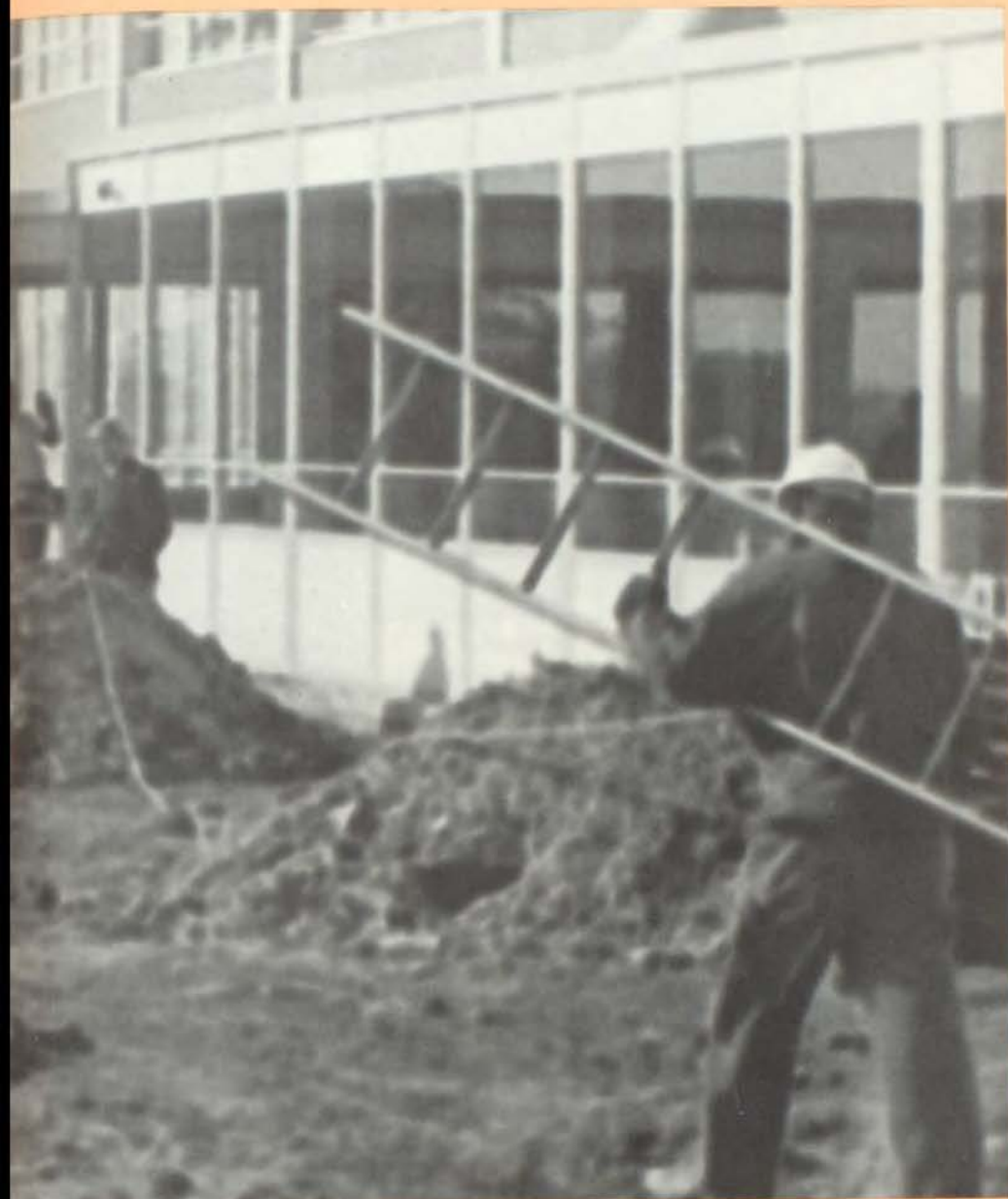
Centerites watch helplessly as workmen destroy the courtyard to make room for the new library.
