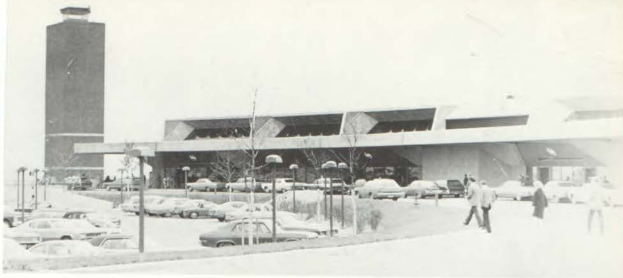
The principal control tower at the new airport looms high over the central TWA terminal building.
