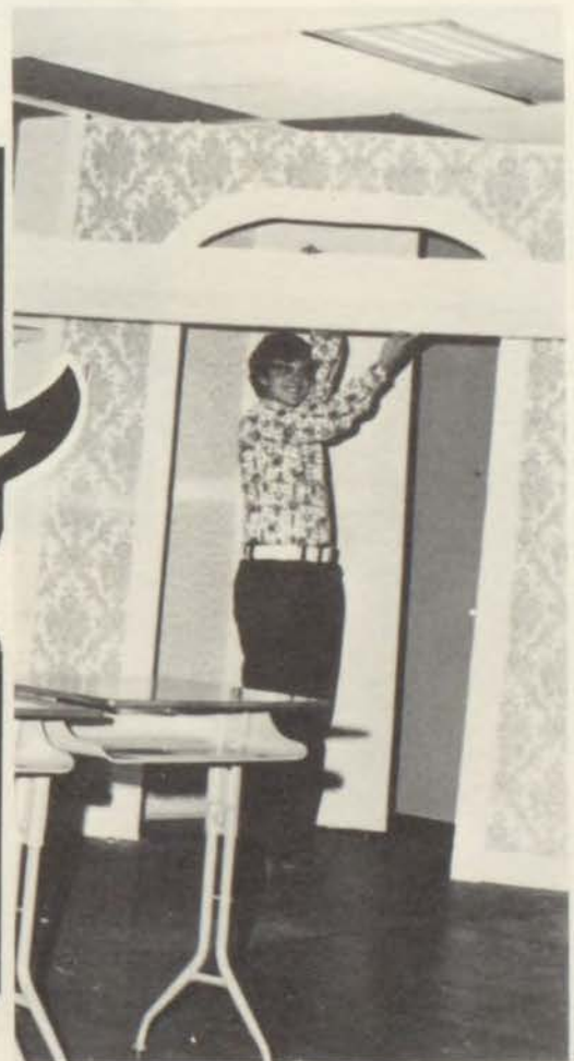
Stage construction keeps Mike Watson busy as he installs styrofoam trim to the set. Mike was an understudy in the play.
