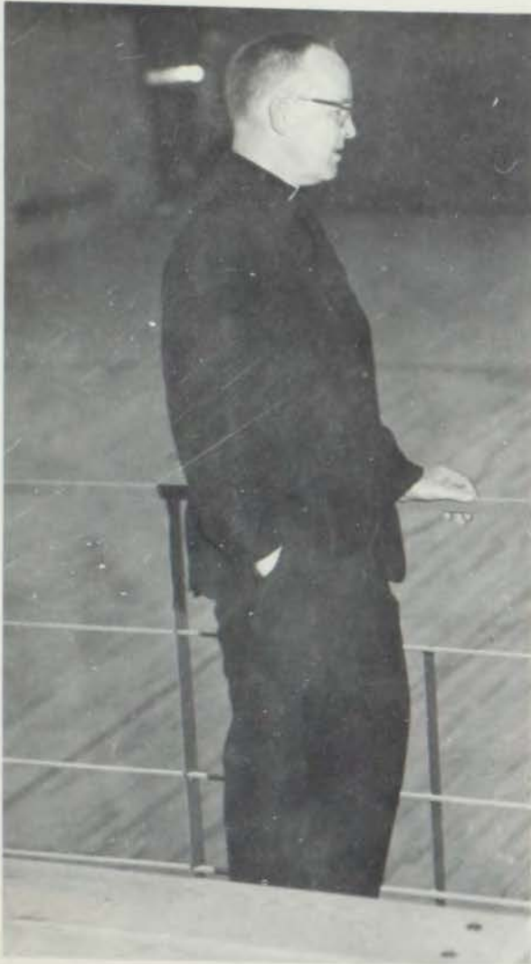
Father Sullivan pauses in a proud mood as he surveys the nearly completed gym.
