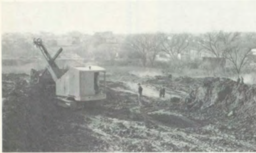
Looking north toward Meyer, bulldozers dig Hogan's basement.
